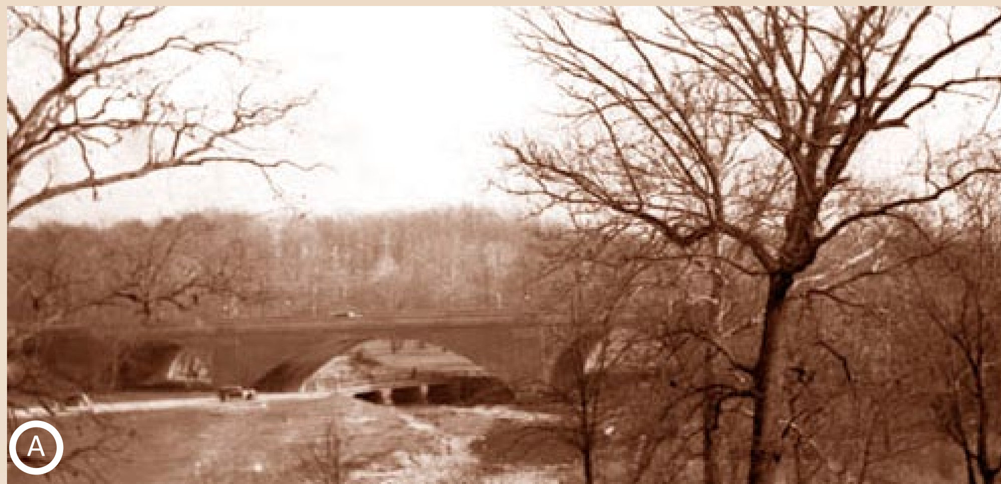
HARFORD ROAD BRIDGE
