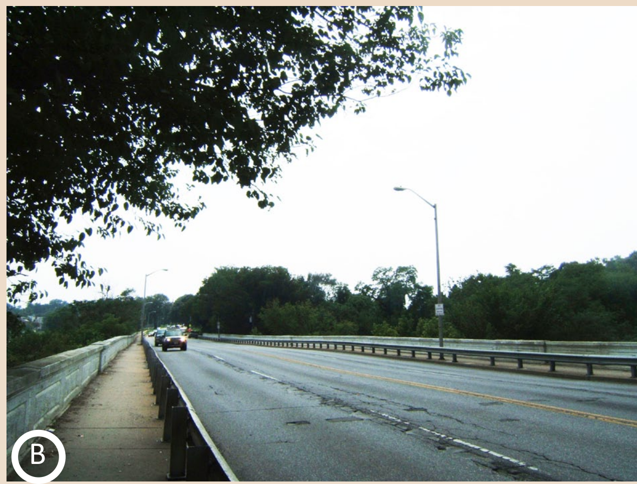
ROAD/WALK OVER HARFORD ROAD BRIDGE
